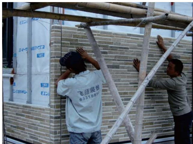
Dry construction method
