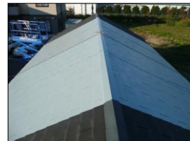
Roof of two rooms are coated with (A) Thermal Barrier Coating (B) Ordinary Paint
