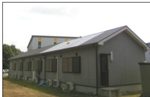
Roof of two rooms are coated with (A) Thermal Barrier Coating (B) Ordinary Paint
